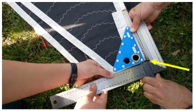
2) Position the head point on top of the clew point and fold the sail along the leech to find the ½ leech point. Put the head point on top of the ½ leech point to find the ¾ point.
